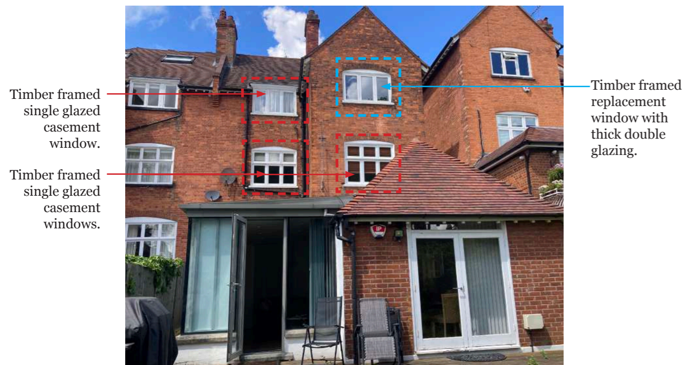
Figure 08: Existing rear elevation.
