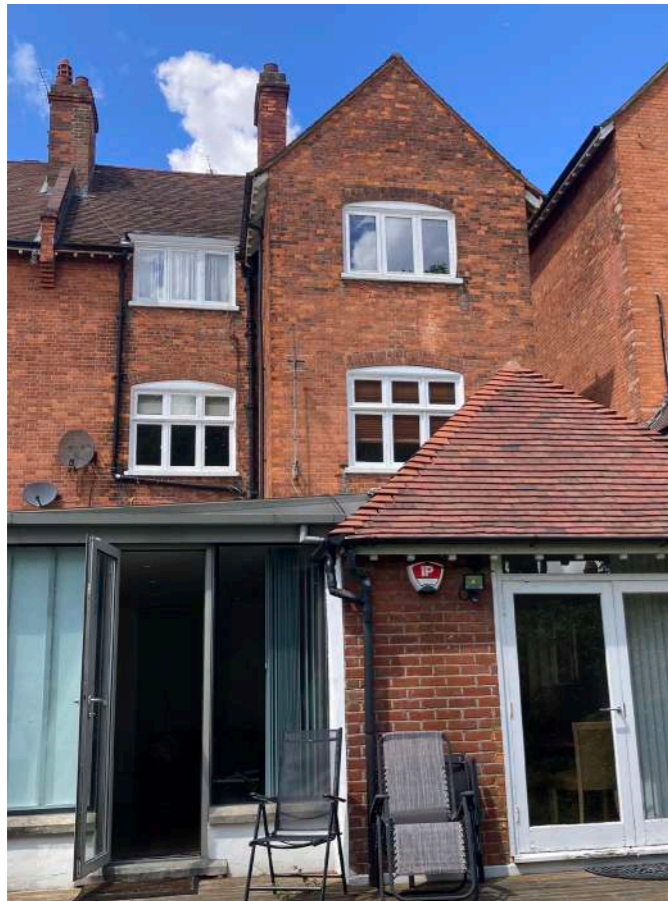
Figure 01: Rear elevation of 25 Oakhill Avenue
