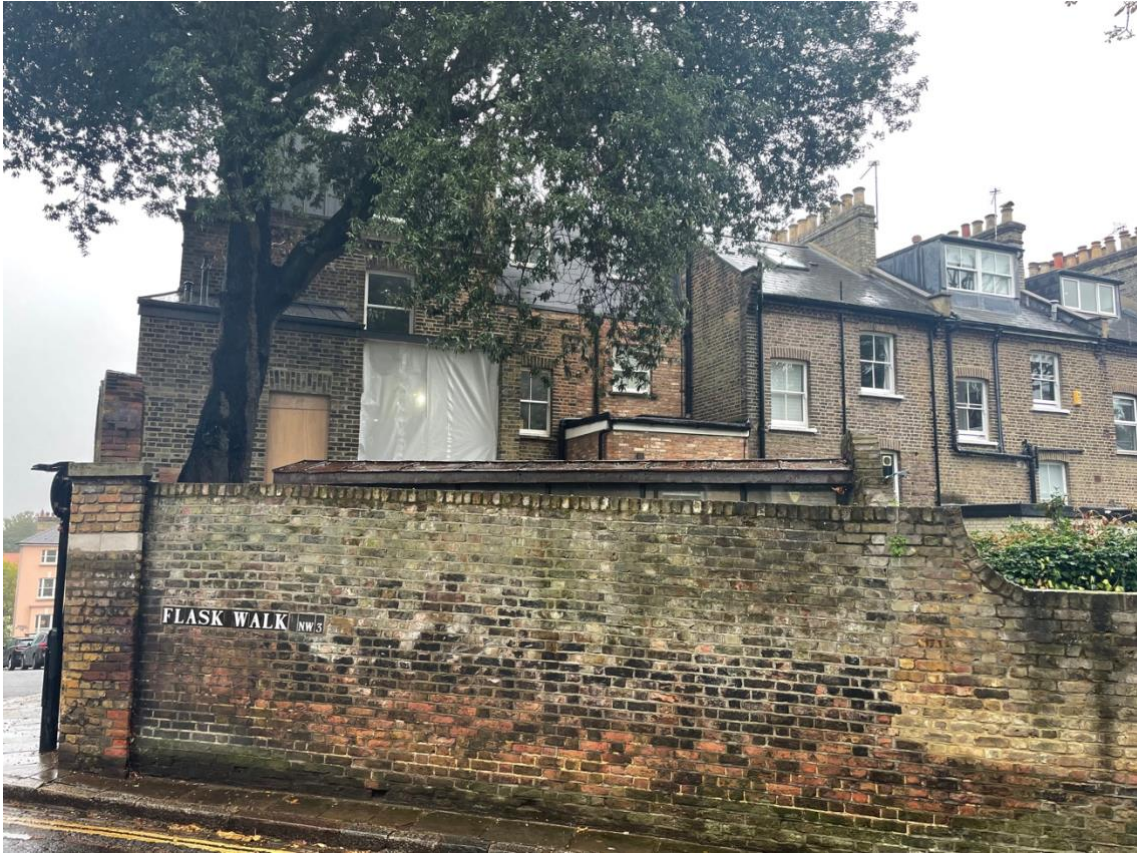
Photo 4: Rear elevation on Flask Walk showing existing pipes on the terrace
