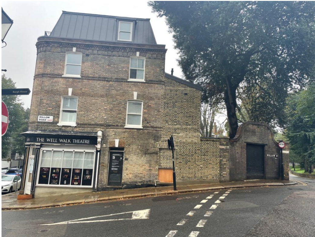
Photo 3: Side elevation fronting Willow Road
