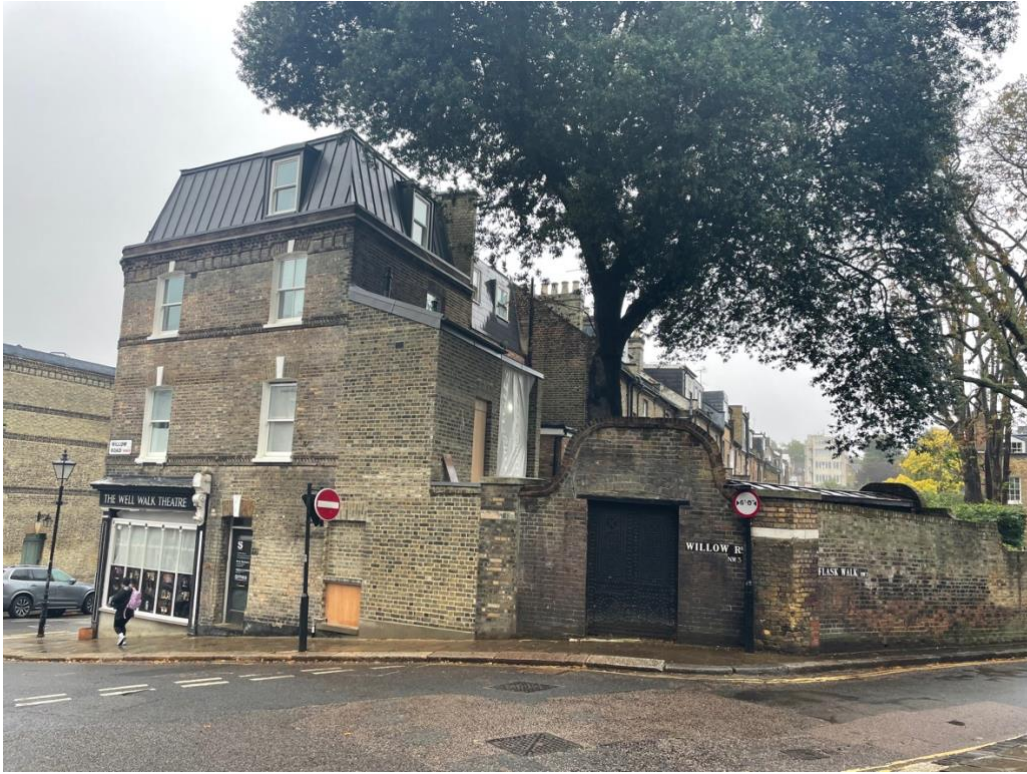
Photo 2: Side elevation fronting Willow Road
