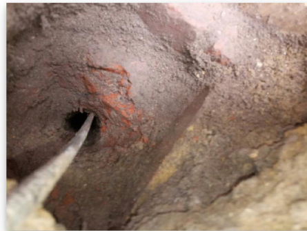
Fig 1.2: Trial Hole 1 Footing
