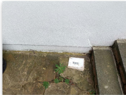
Fig 1.1: Trial Hole 1 Location
