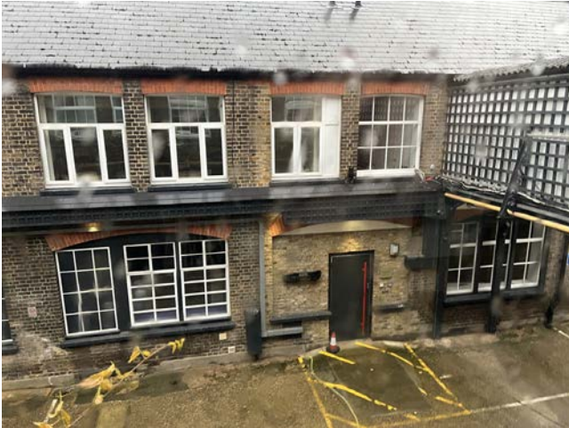
Plate 3 View showing disjointed appearance of windows to historic structure and blocked up former opening to centre. Note also poor appearance of link bridge.
