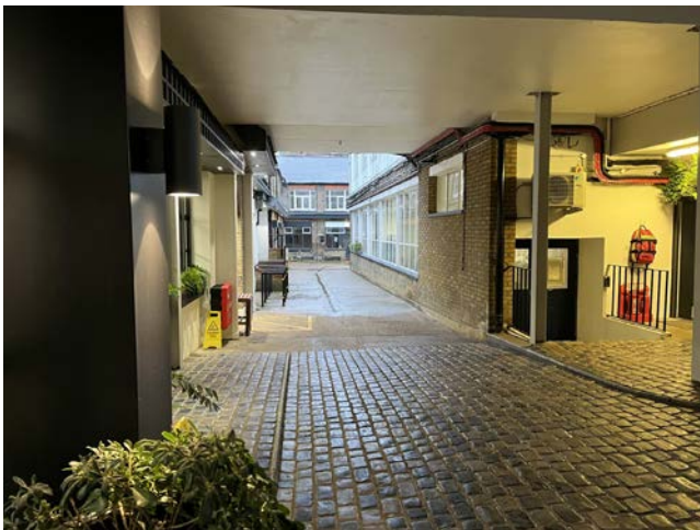
Plate 7 View looking east from within the north western section of the building. Notice almost all structures visible are mid 20th century. Flooring here features granite setts that replaced concrete hardstanding in the 21st century.
