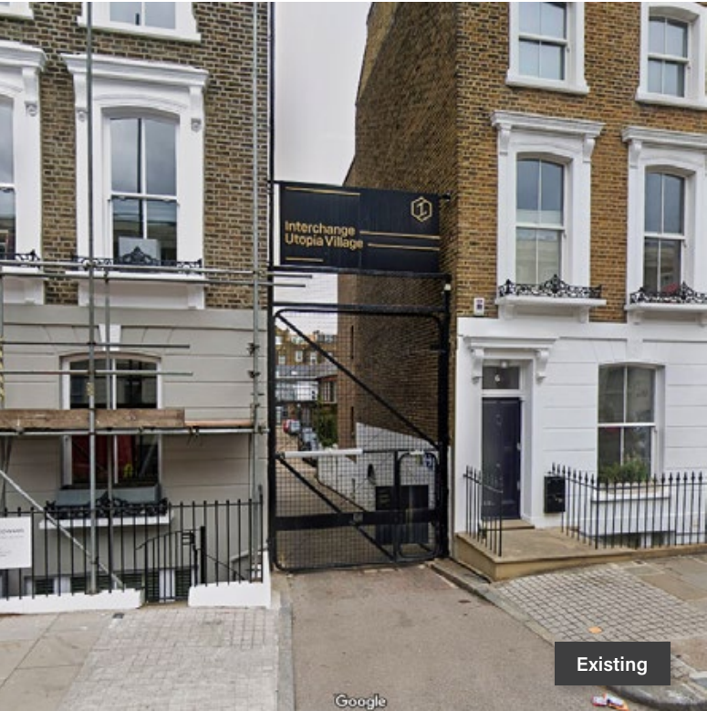
Entrance Gate – Chalcot Road
