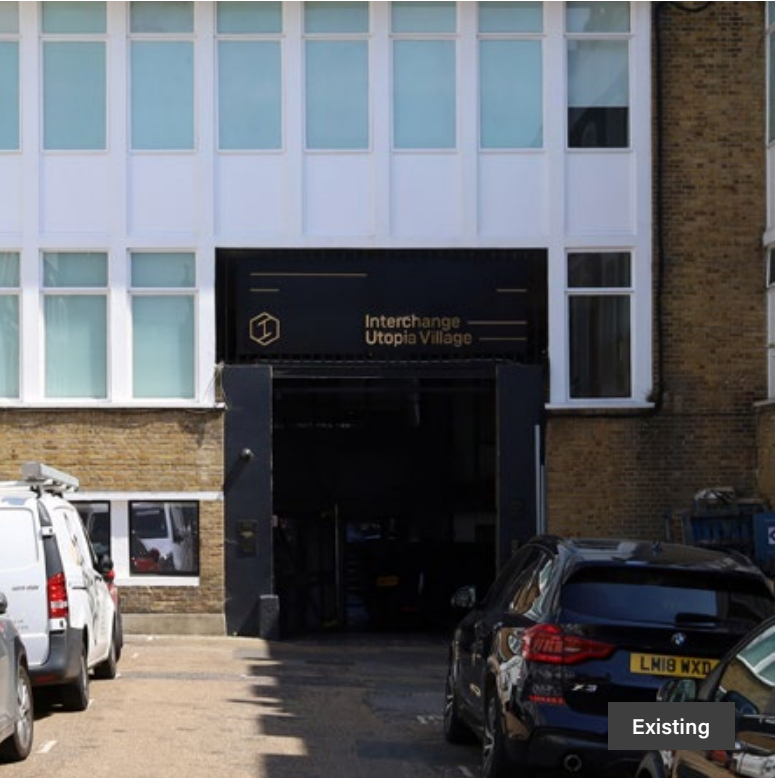
Entrance Gate – Chalcot Road
