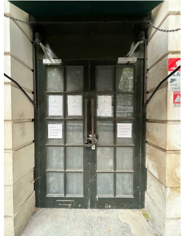
Existing Entrance Door and Awning
