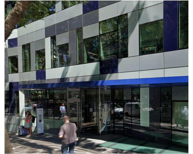
Fig. 2.1b - ARUP Fitzroy Street
