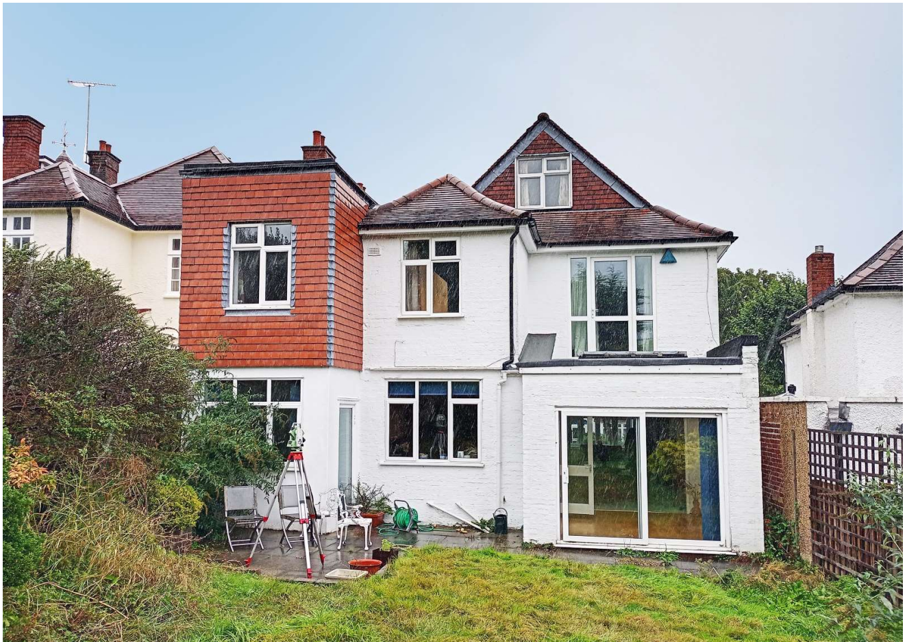
Figure 7 - Existing photograph of the rear façade
