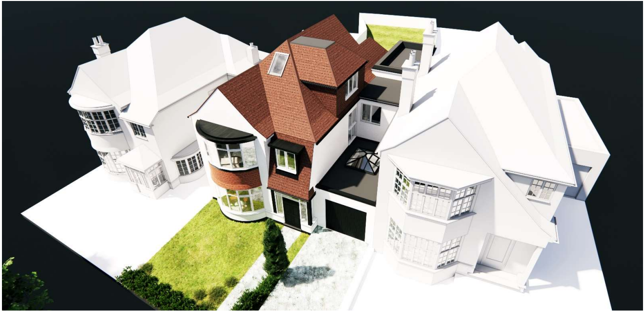
Figure 11 – Illustrated aerial view of the front of the property showing the massing of the mansard dormer and the lantern rooflight over the study.
