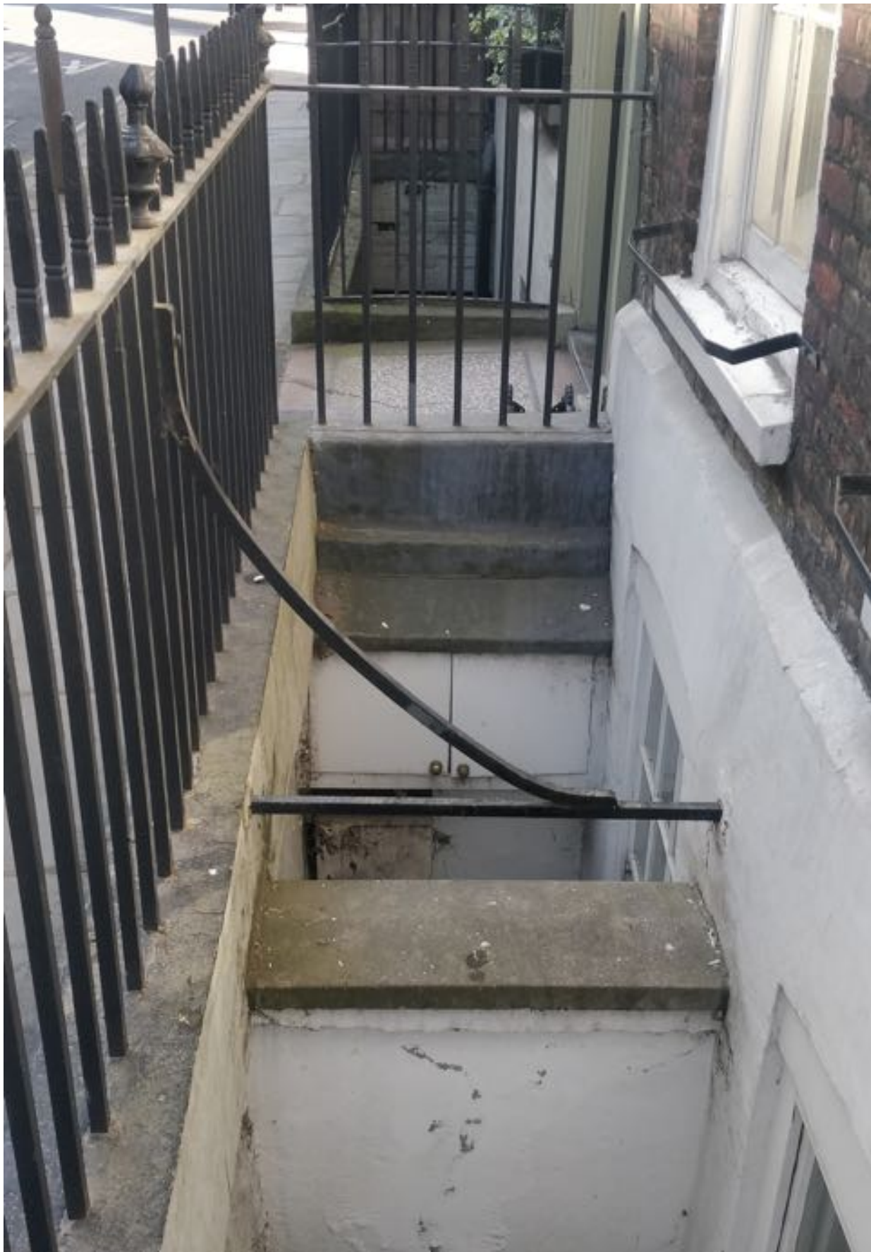
Current design of railing brace at 37 Great James Street. Proposed to be replaced to allow for greater headroom over stair
