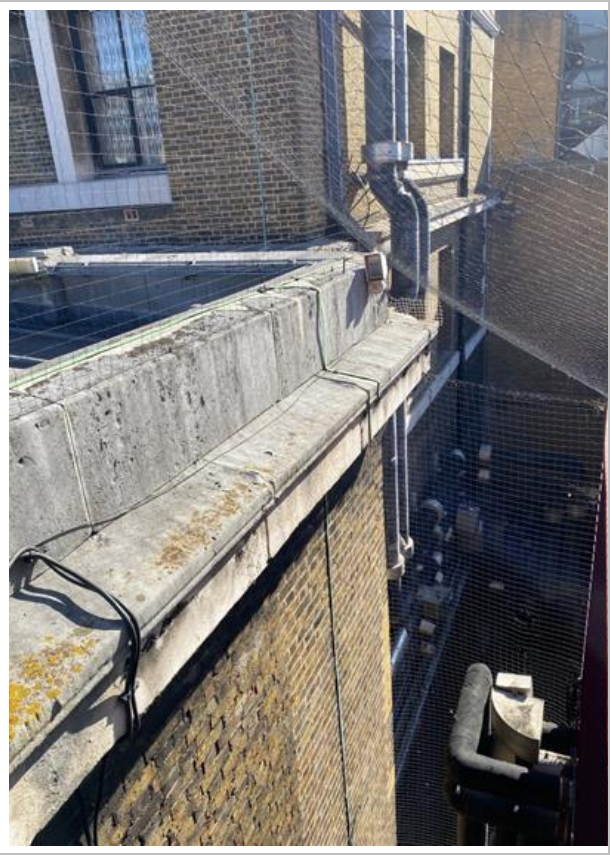
Photo 2 – Showing netting in place at top of fire well escape of the brick built energy building
