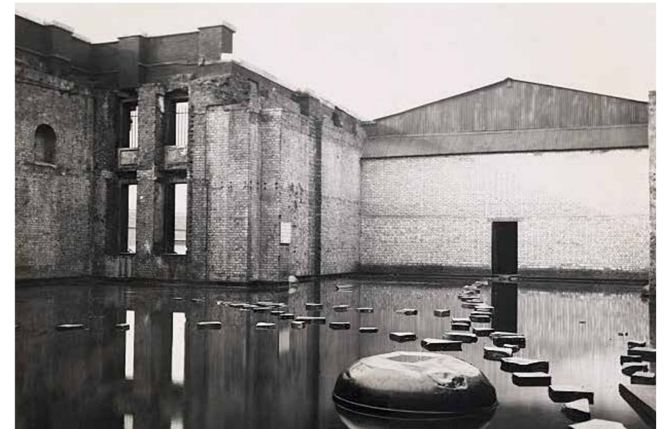
Figure 3.2 Post-war photograph showing damage to the Lycian Building
