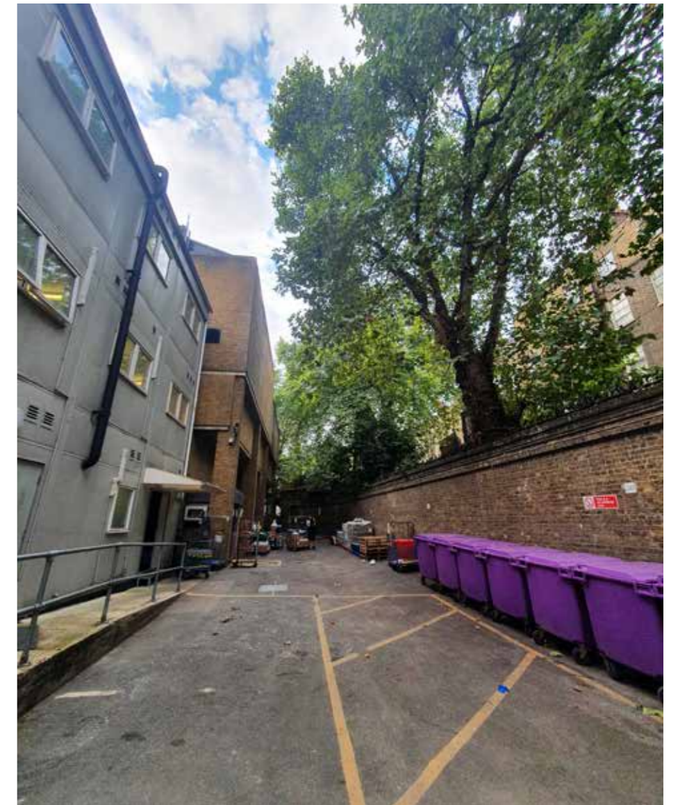
Figure 3.8 The portacabin block which adjoins the northern elevation of the New Wing
