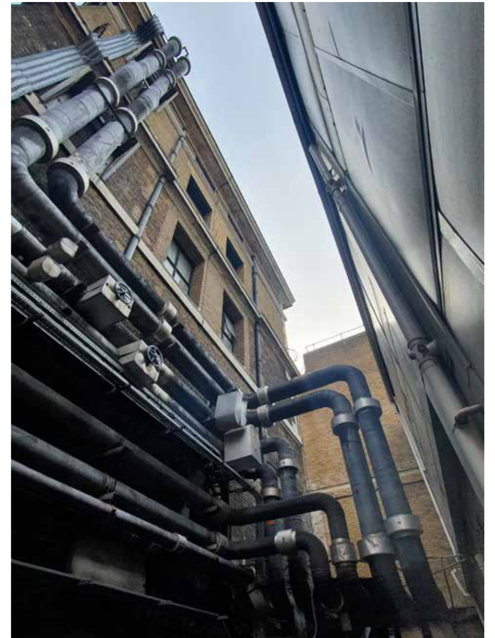
Figure 1.6 The west elevation of the Lycian gallery
