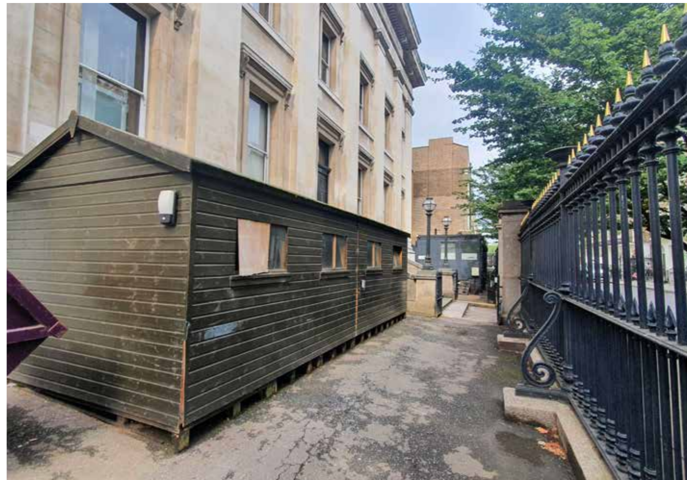
Figure 1.8 Portacabin to the east elevation of the White Wing, ISS site
