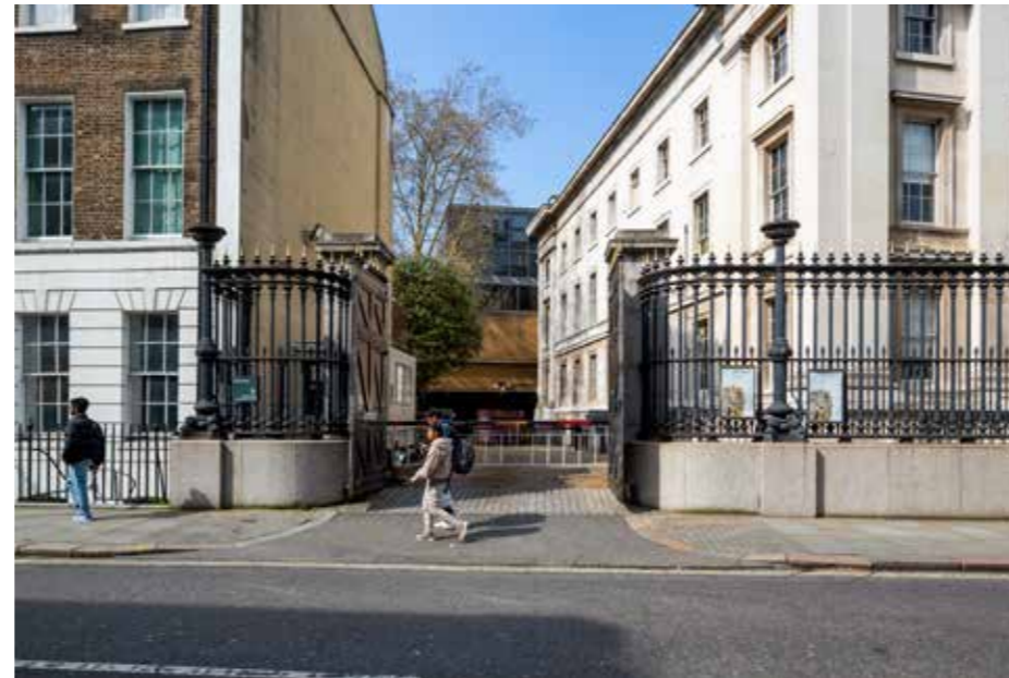
Figure 3.15 View into the service areas of the Museum Estate to the rear of nos. 89-91 Great Russell Street. The SWEC site lies beyond the New Wing.
