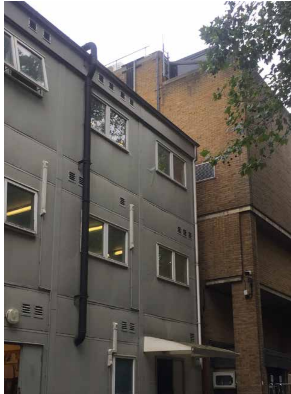
Figure 1.5 The existing portacabin block
