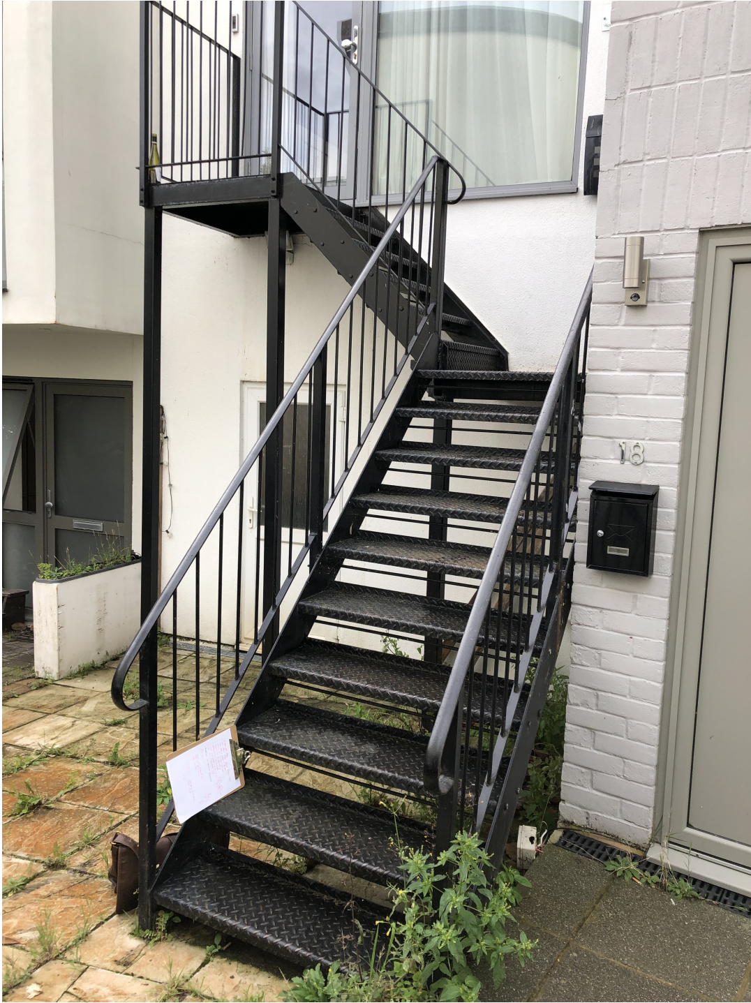
Rear access staircase
