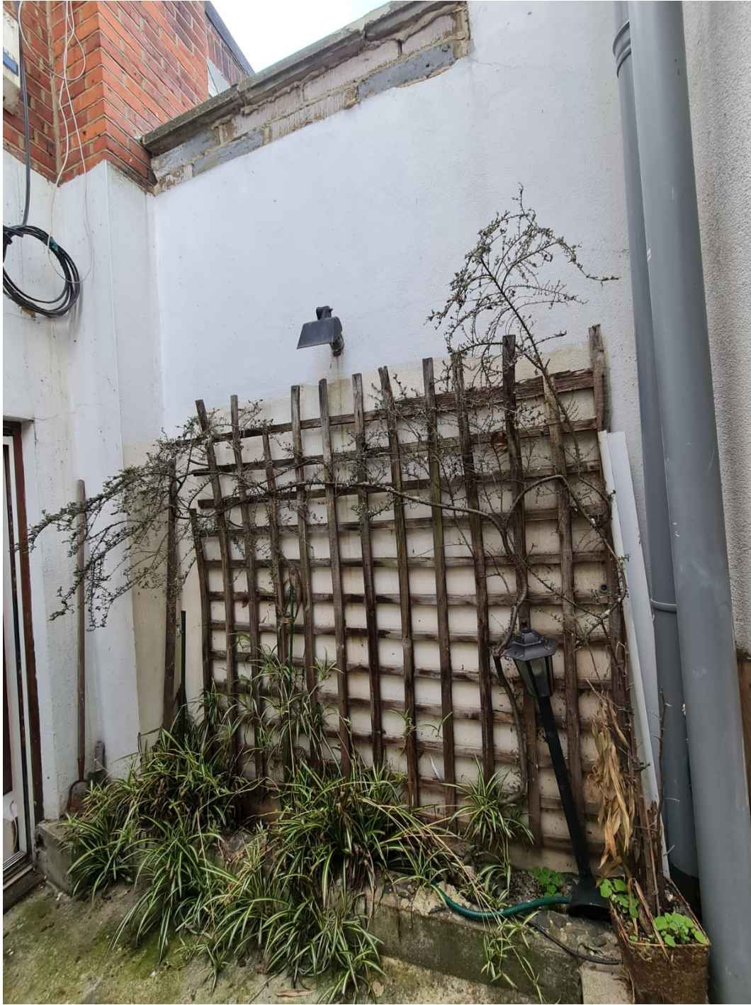
Rear courtyard looking north
