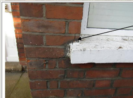
Photograph 5 front RHS bay
