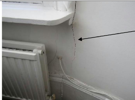
Photograph 14 Front LHS bedroom – below bay window
