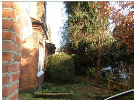
Photograph 11 front PH and TP vegetation
