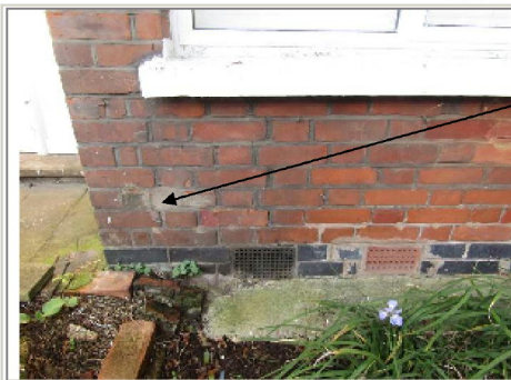
Photograph 4 front RHS bay
