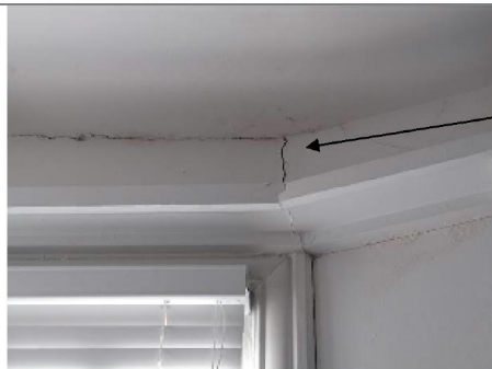
Photograph 15 Front LHS bedroom – above bay window
