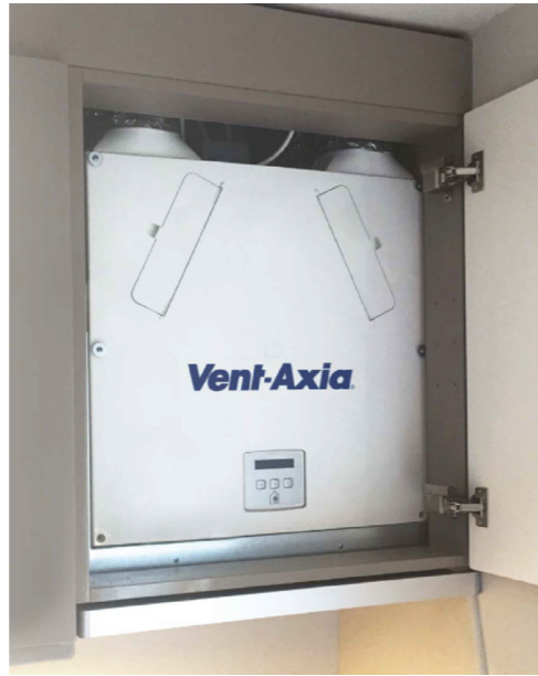
MVHR Unit Installation Example
