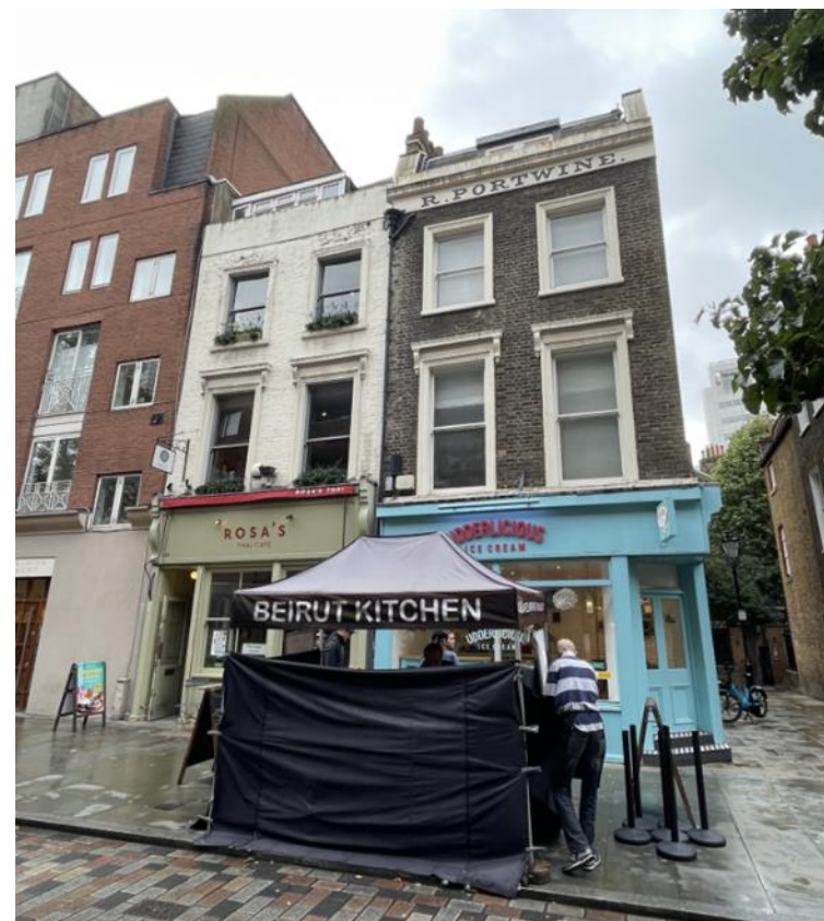
Plate 6: 24 and 26 Earlham Street, front elevation.
