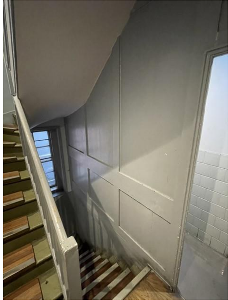
Plate 11: Timber panel partition on second floor.
