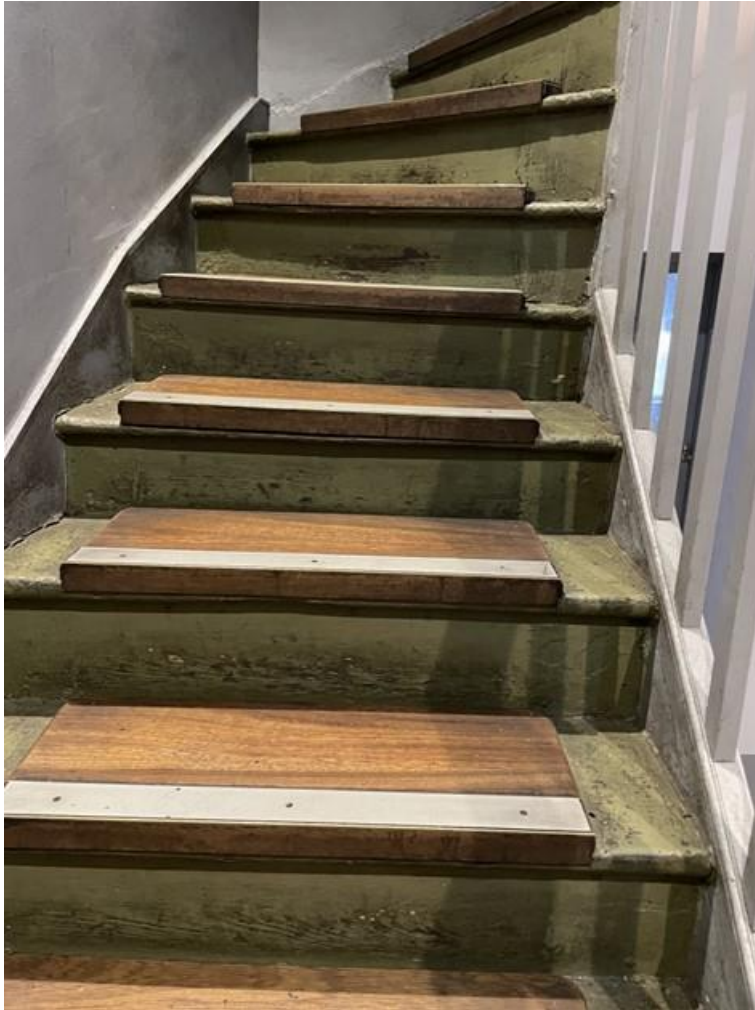
Plate 10: Historic staircase with modern coverings.
