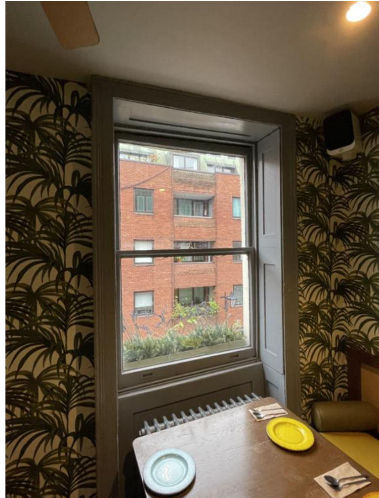
Plate 9: Timber-framed window and bay at the second floor, including original shutters.
