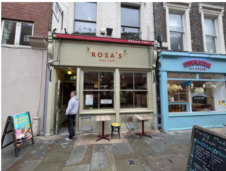
Plate 7: No. 26 Earlham Street shopfront (the site).
