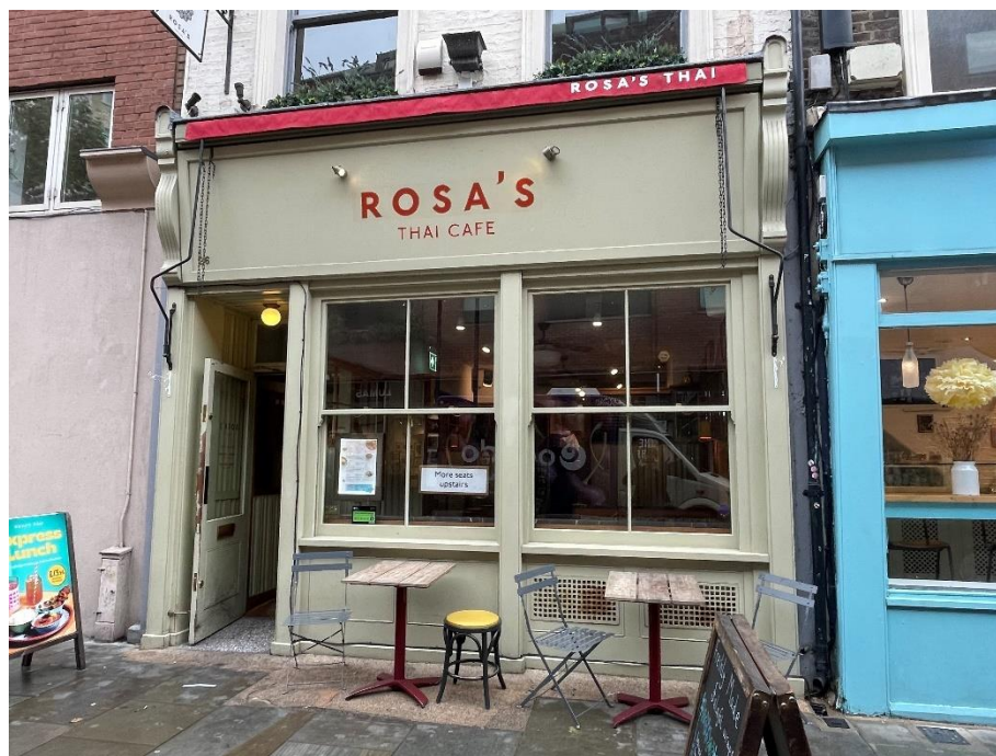
Figure 1: Application Site (Front)
