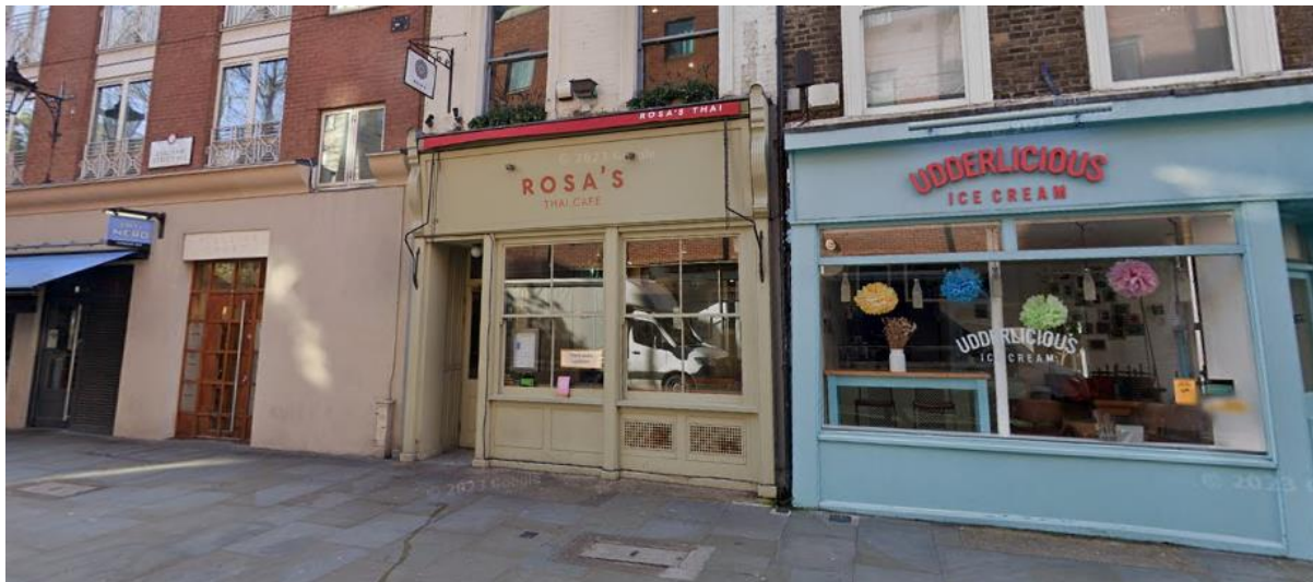
Figure 2: Application Site (inc. ground and first floor frontage) with Fielding Court entrance (left) and Udderlicious (right)
