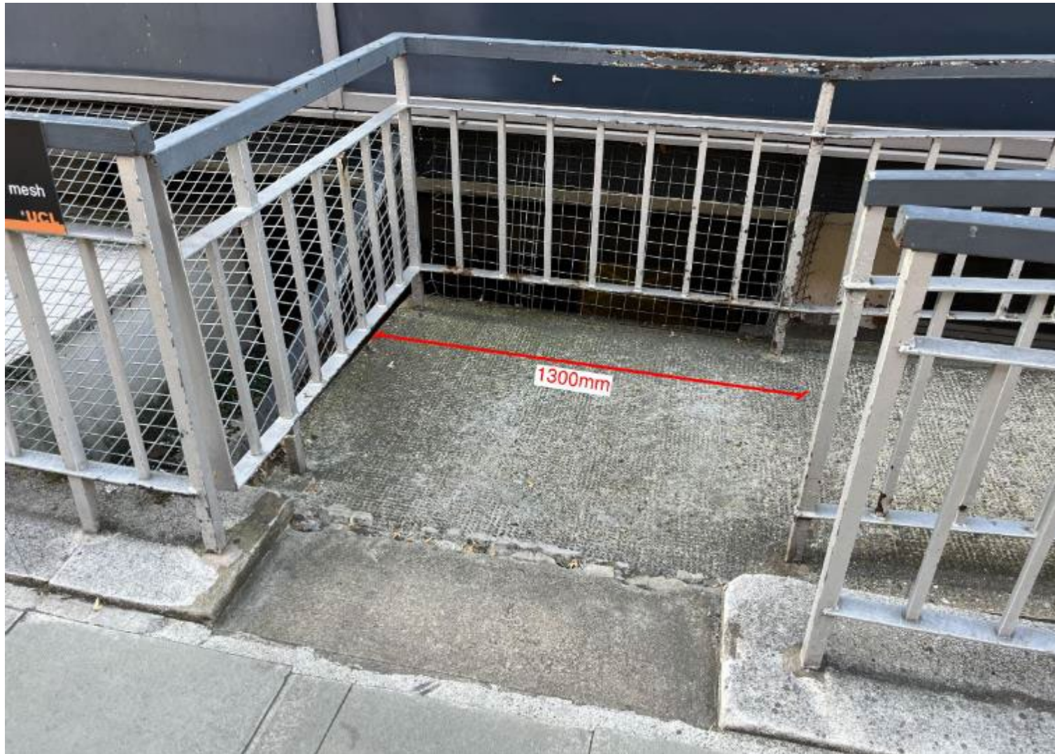
Figure 3. Indication of the current clear width of the bottom landing of the ramp (in red).
