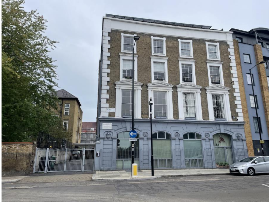
View of the new gates from York Way in the current building setting
