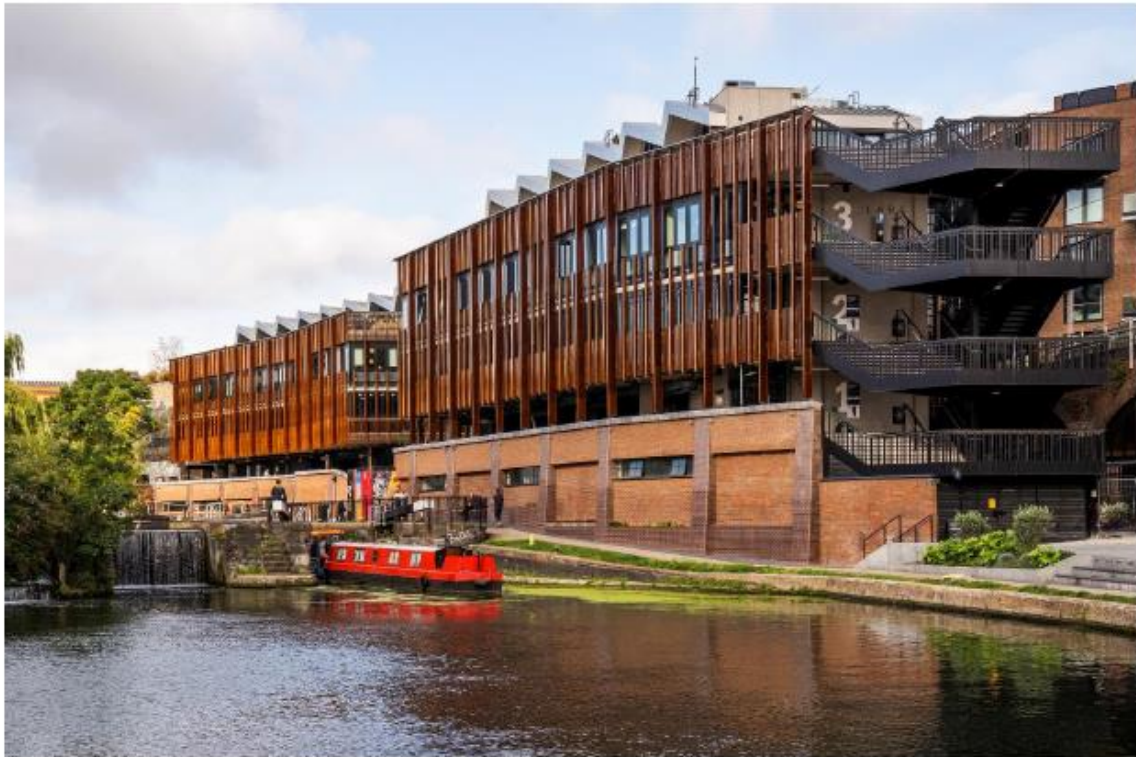
Unit M100, Hawley Wharf, Camden
