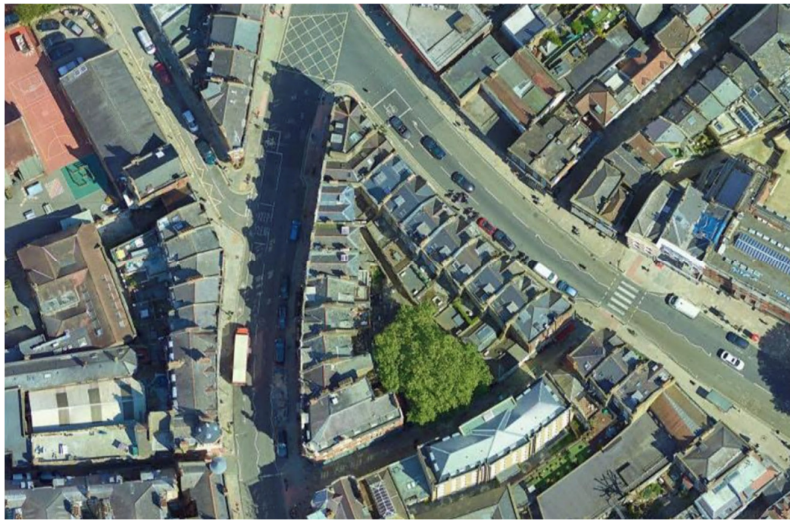
(Aerial view of 30 Heath Street and surrounding buildings)
