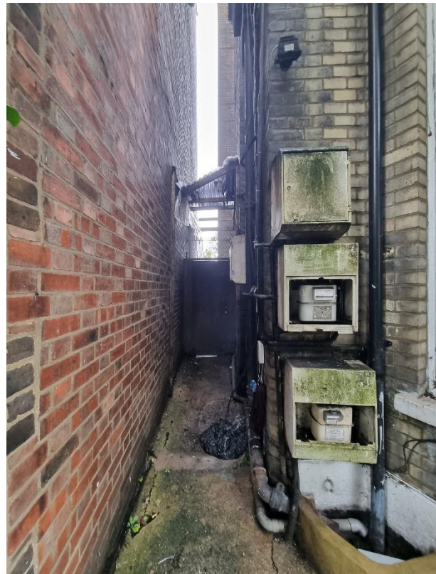
Fig 2 – View through side access and existing gate to be retained
