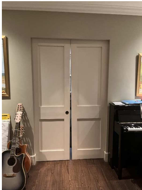
Image 16. Sliding door opening with new 'pockets' built on rear room side.
