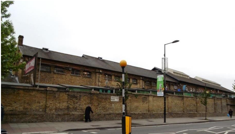
Figure 4.1: View of Horse Hospital and boundary wall from north on Chalk Farm Road
