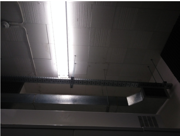
Existing ceiling tile finish with surface mounted ductwork
