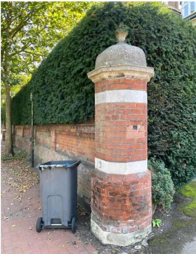
11. West Heath Road pier (East)
