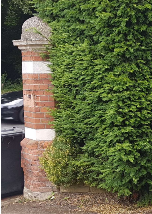
12. West Heath Road pier (East), damaged and spalled brickwork
