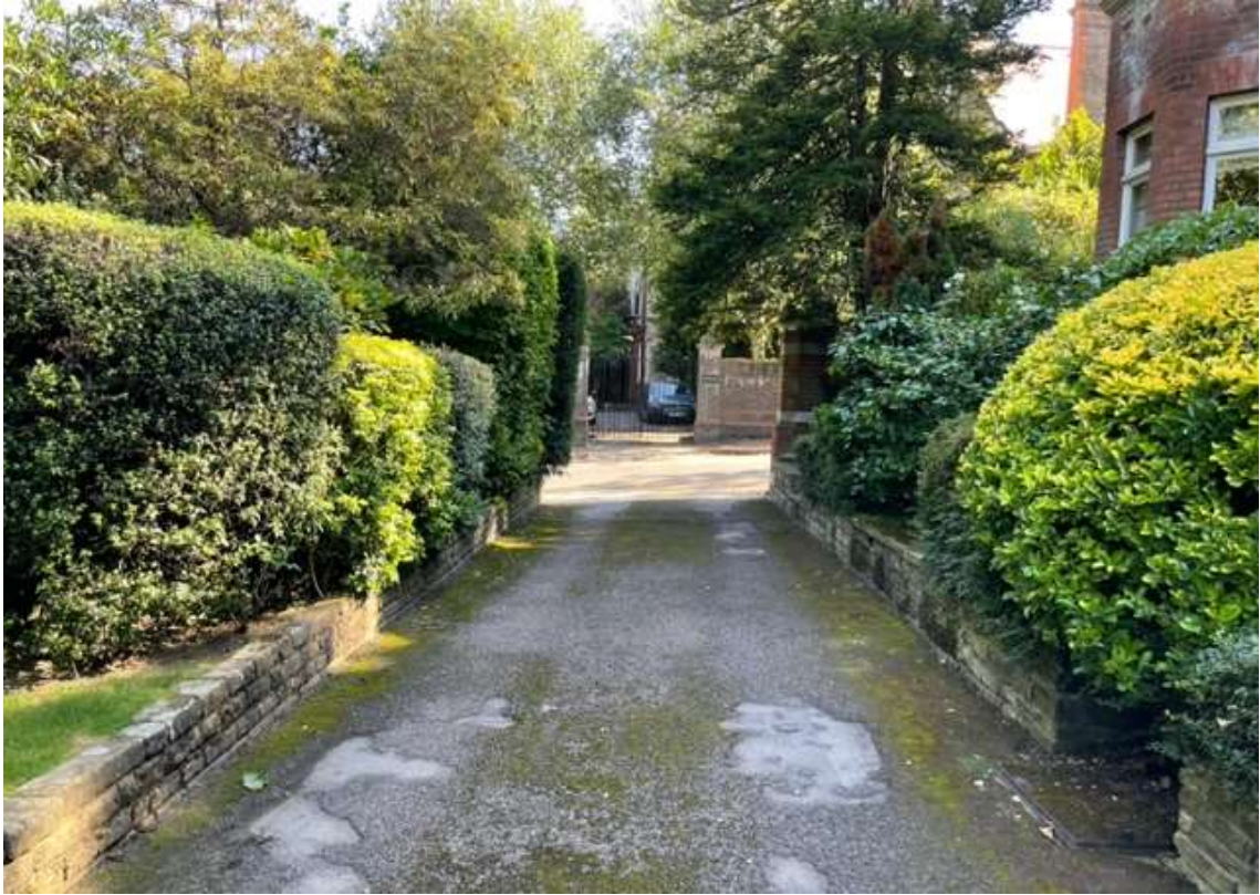
10. Driveway, looking towards Redington Road
