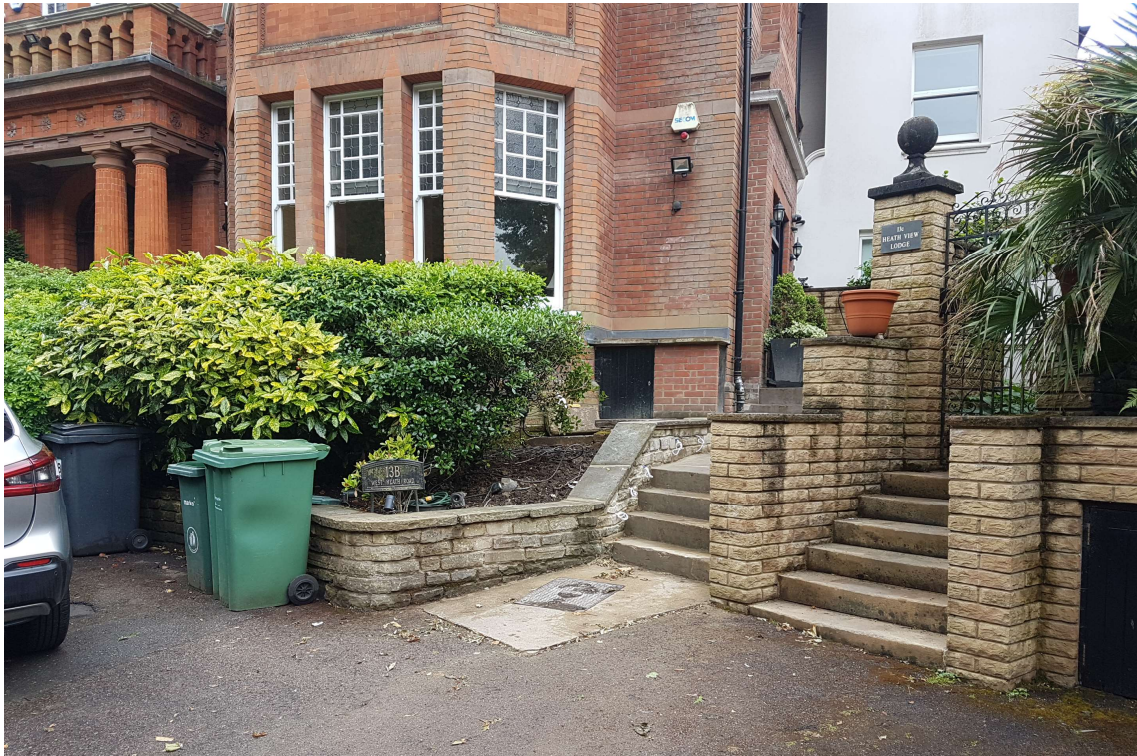
14. Existing internal stone walls and pavings
