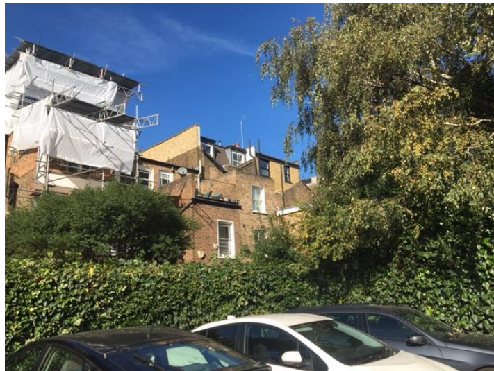
Rear elevation of Gayton Road terrace showing the degree of existing alteration
