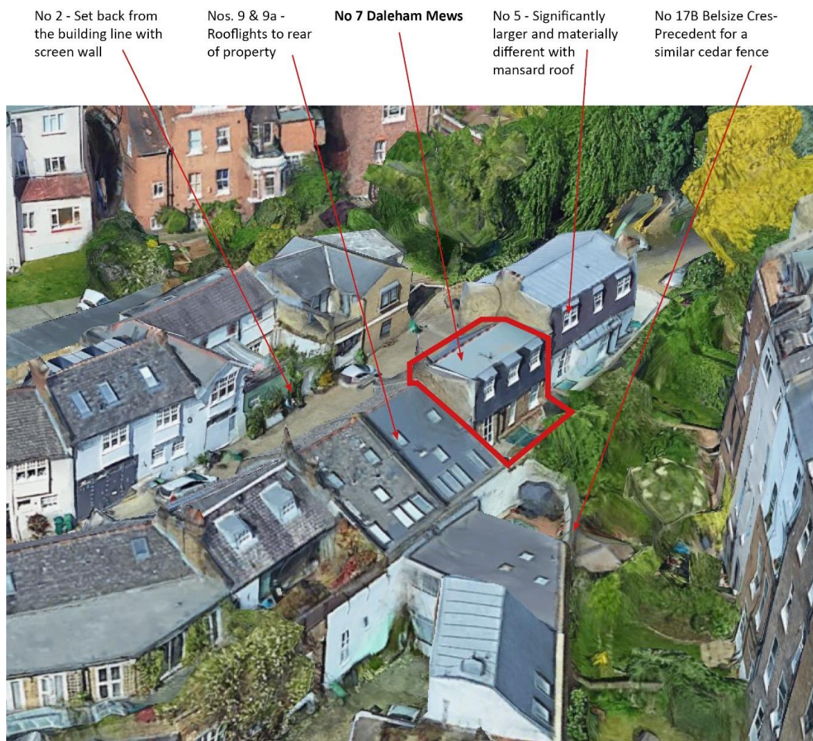
Figure 3. Aerial view of the rear of the properties looking North West
