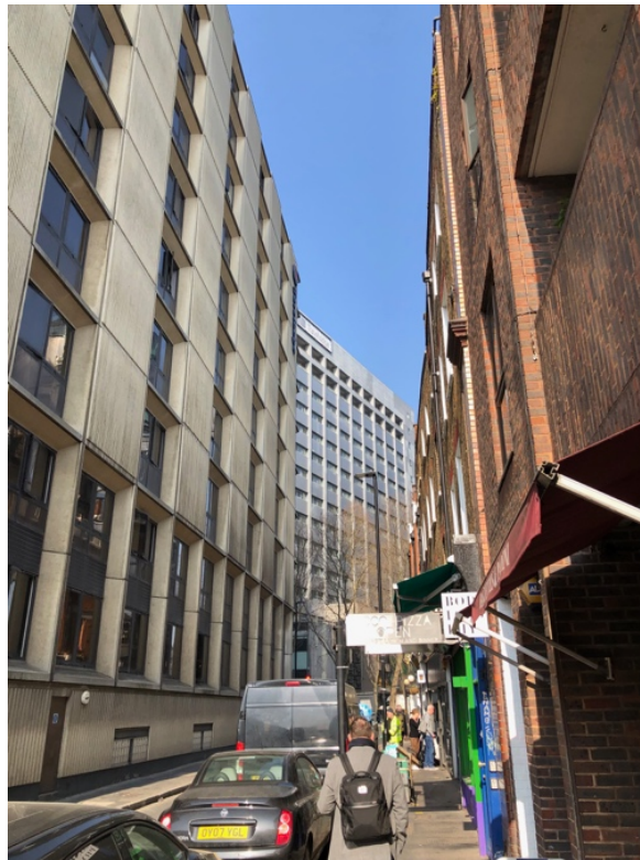
The existing view from the western pavement of Drury Lane with the Selkirk House/Travelodge building beyond.
