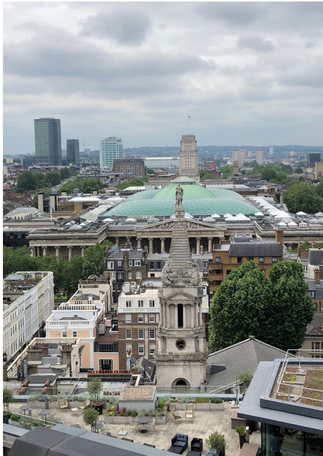
The view looking north showing the close proximity of the neighbouring Grade I listed buildings of St George's Bloomsbury and the British Museum.
