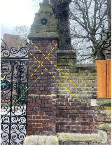
6No.Cross Stitching/Pinning of Cracks to each pier: Mark out and agree with engineer positions of X pinning dependent upon expected depth of ties. Drill 18mm Staggered holes approx. 300 mm crs apart. Drill 18mm holes approx. 1250mm deep. Insert 10mm stainless steel tie and fully back-grout. Leave tie below the finished surface ready for striking off and plugging with clear resin mixed with brick dust polished flush to brick face.
