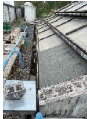
Roof Paving Slabs And Roof Lights damage
