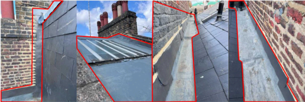
Schedule A Item 4 – Waterproof membranes/linings currently present on the roof are not limited to these photos.
