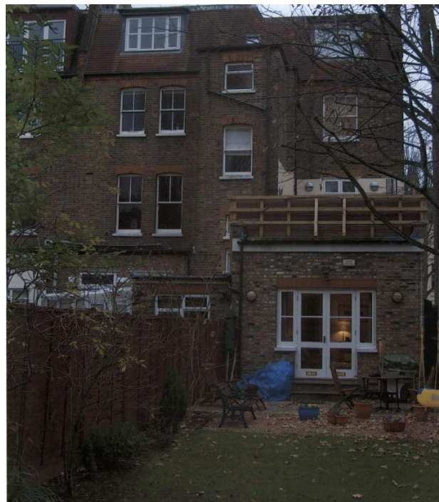
Figure. 6 shows Flat 1 and 2 Greencroft Gardens and the pre-existing conservatory extension
