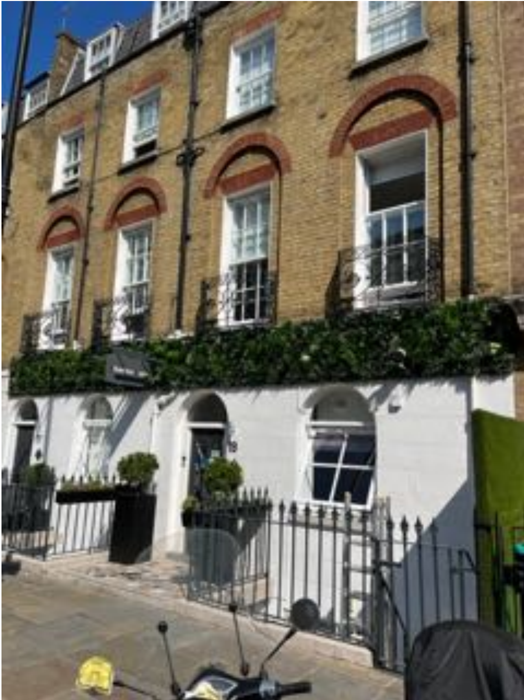
Image 03 -Front Elevation after the installation of the plant panel - Alhambra Hotel in centre.
