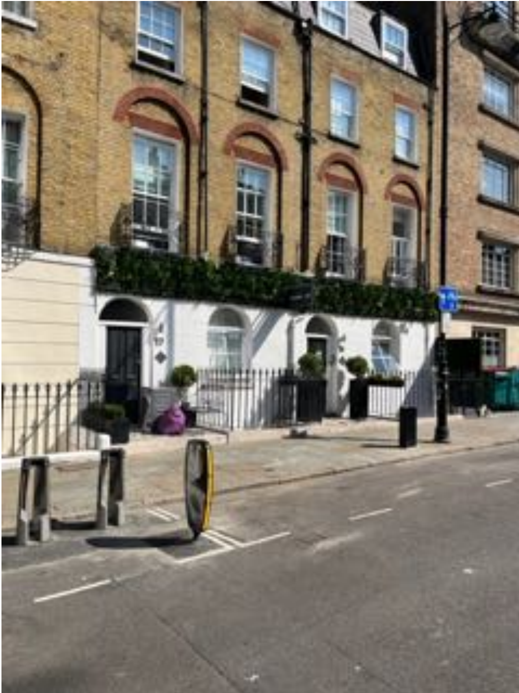
Image 02 - Front Elevation after the installation of the plant panel - Alhambra Hotel in centre, No15 to the left, Derbyshire House to the right.
