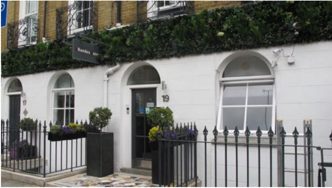
Image 04 - Front Elevation detail after installation of the plant panel.
