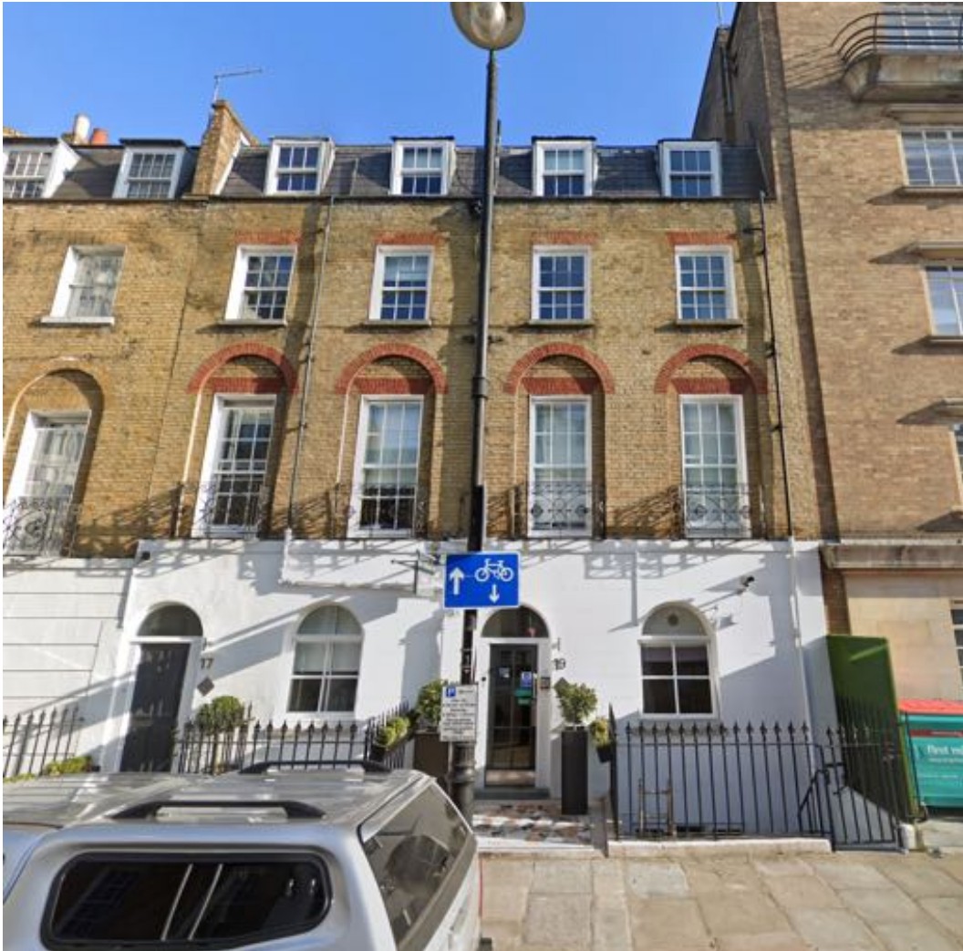
Image 01 – Front Elevation before the installation of the plant panel - Alhambra Hotel in centre, No15 to the left, Derbyshire House to the right
