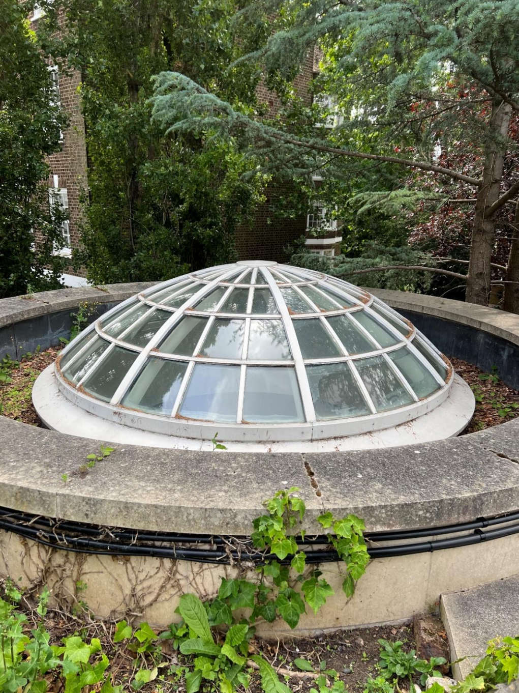
Existing domed rooflight to be replaced.
