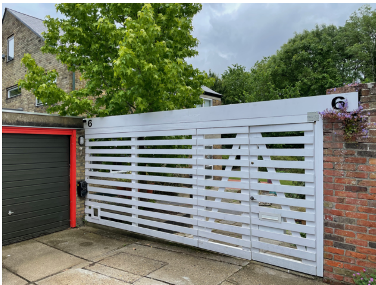
PHOTO 1: EXISTING TIMBER GATE NOT TO SCALE
