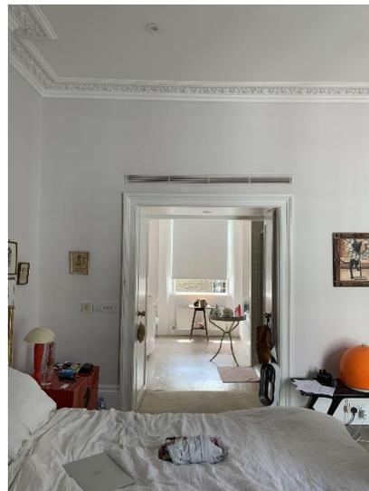
Figure 21: The modern opening in the spine wall at 2<sup>nd</sup> floor level.
