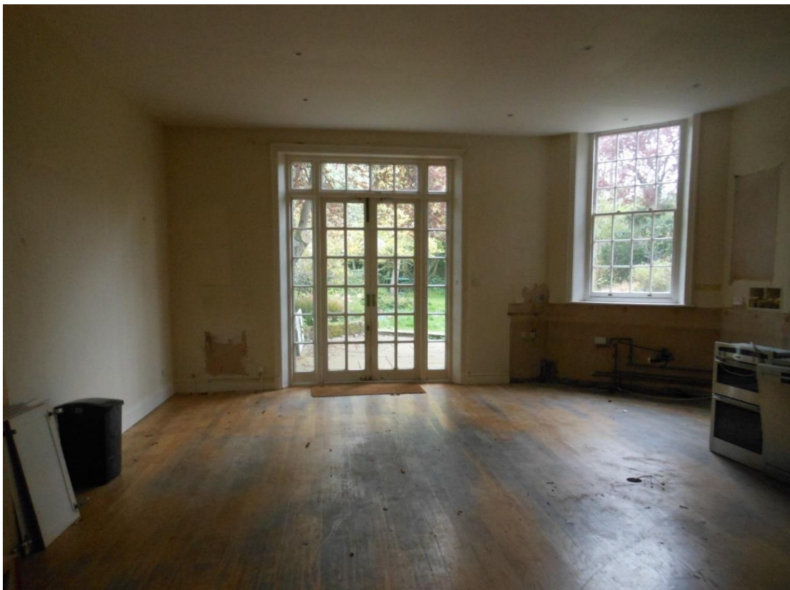
Fig. 10: The former studio looking north-west towards the garden (24 April 2023). In the 1960s the windows and doors were removed from the two openings to create a loggia open to the garden. Windows and doors were reinstated in the 1990s.
