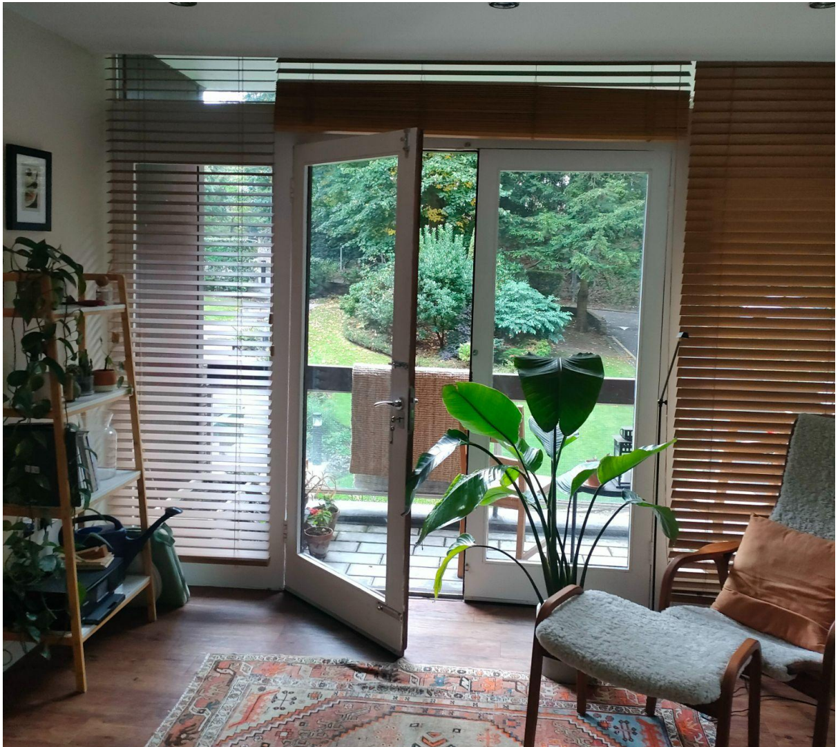
Image 7. Existing wooden balcony doors, from inside.
