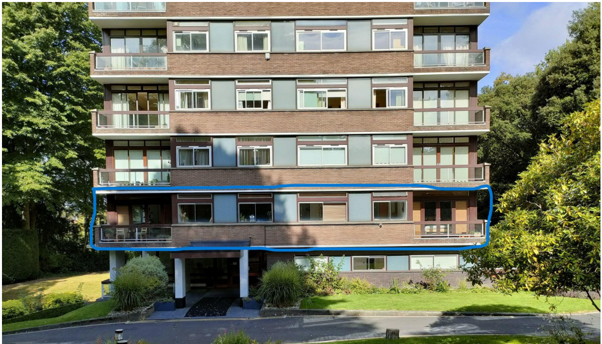
Image 2. View from the front garden, with apartment windows and balcony doors highlighted in blue.
