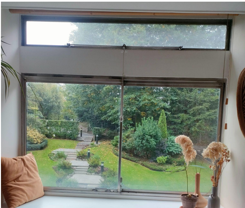
Image 5. Existing frames, from inside - sliding panes with upper tipper casement.
