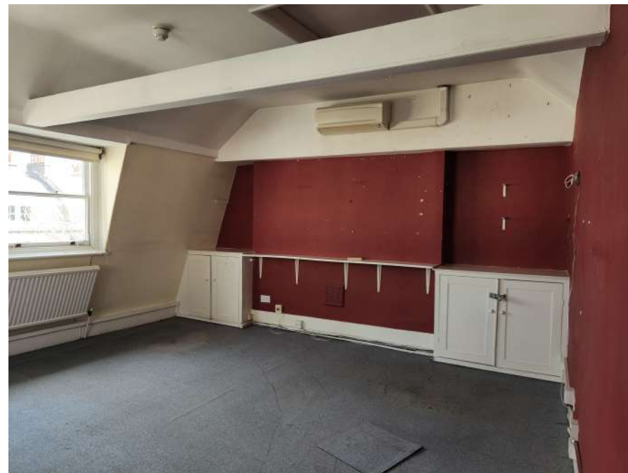
Figure 27: Third floor NB ceiling raised and tie beam of truss boxed in.
