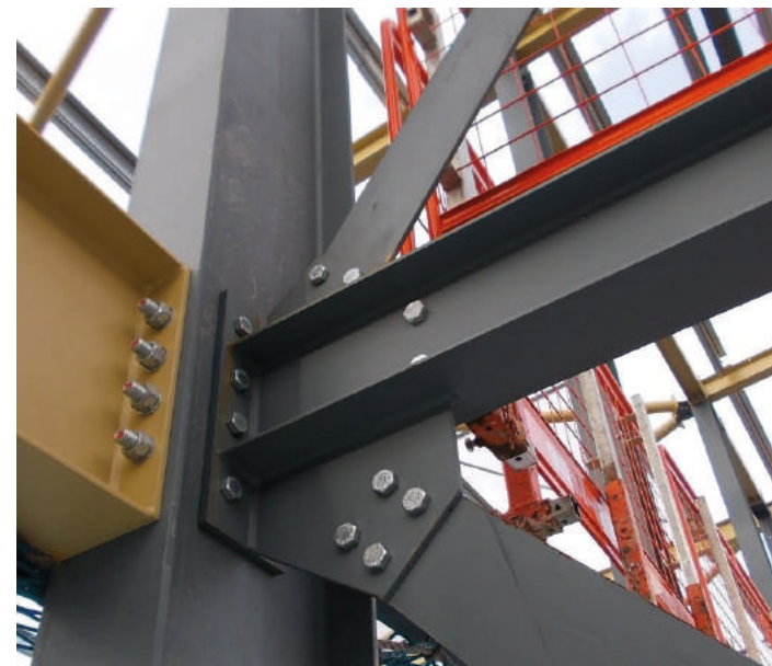
Figure 8.3: Bolted steel connection
