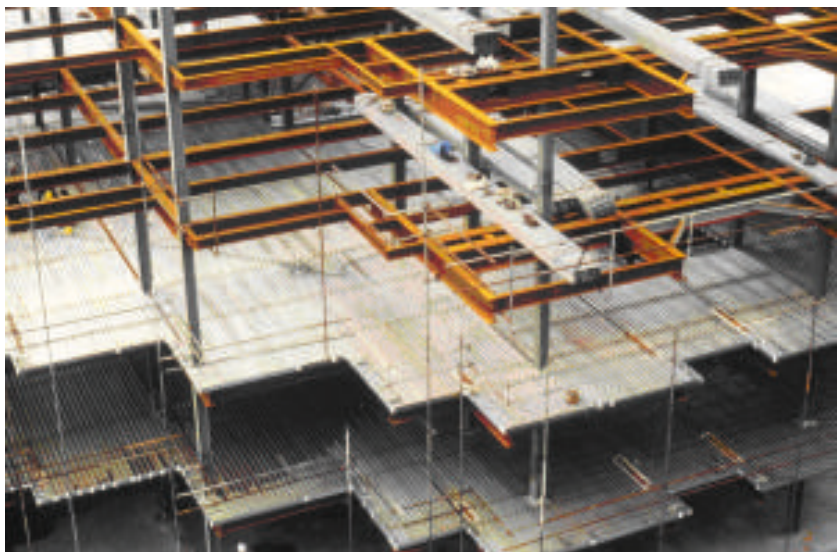
Figure 9.1: Plan of proposed structural solution (top right), section indicating where RC frame would change to a steel frame (bottom right) and example of hybrid steel and concrete frame structure.
