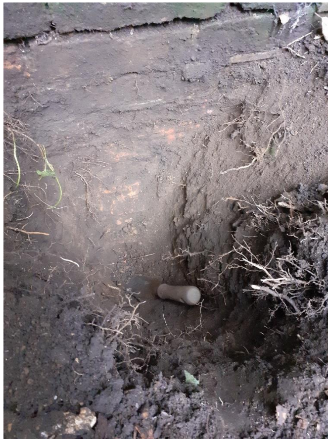
Photo 12 of the depth of the wall foundations – roots were from on site ivy which has been mostly removed
