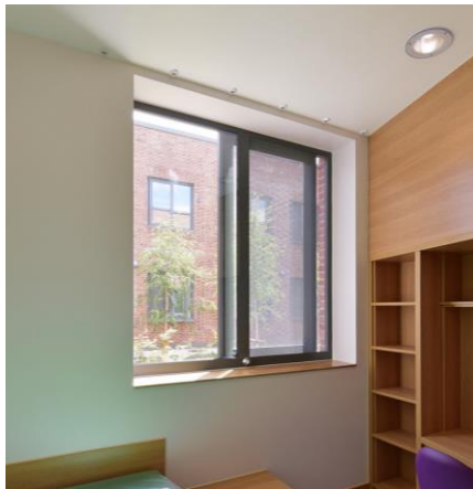
Above: example of horizontal sliding window designed for mental health environments, internal and external view, illustrating transparency of steel mesh. N.B. Proposed colour is white
