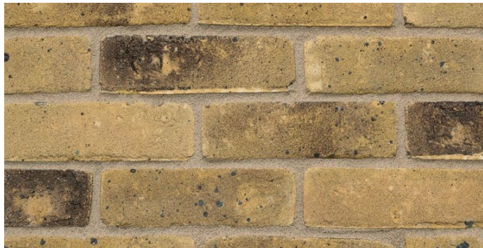
Existing Yellow London stock brick facade
