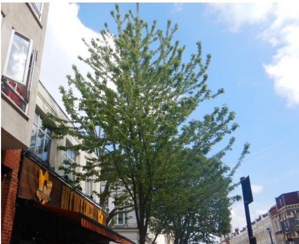
Showing encroachment of T1 onto the building
