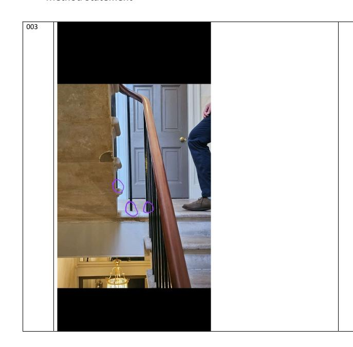
We will also remove the lead from the stanchions that have been circled and install resin to lock them into position and repoint above the resin using a Portland repair mortar.
