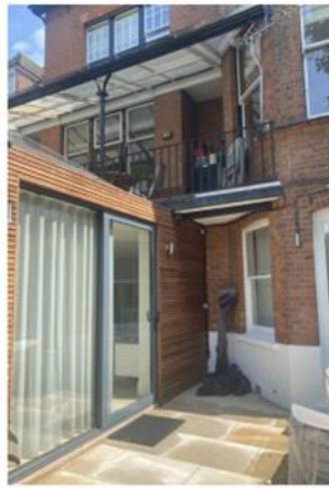
B: Existing lower ground floor rear extension to be replaced
