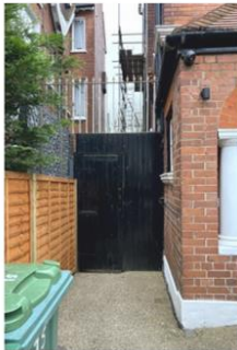
A. Existing timber side access to Flat 1 and Garden
