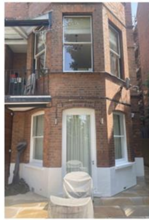
C: Existing rear bay window
