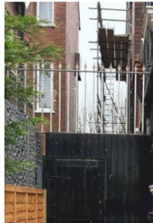
B. Screen and door formed in black painted timber panels with decorative metal spikes above
