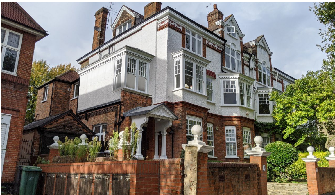
Proposed view of 9 Heath Drive with 1 st floor side extension as per the pre-planning advice
