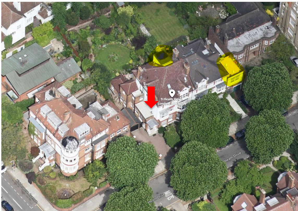
Aerial view of the site
