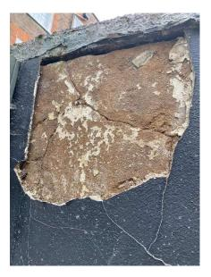
2.7 This is exacerbated by the raised ground level against the wall at 98. The tree has pushed the wall over so the copings are out of line and showing a bow in the wall. Rectification required after party wall agreement in place. It is proposed to put back exactly as it was, with lime based or similar compatible rendering.
