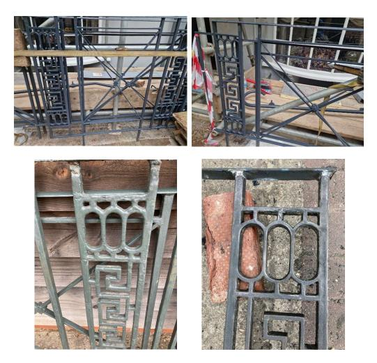
2.10 Finally, it is proposed to replace the metal panel that is attached to the rear of the railings to the front which is rusted with a new one. Again a like for like replacement is proposed.
