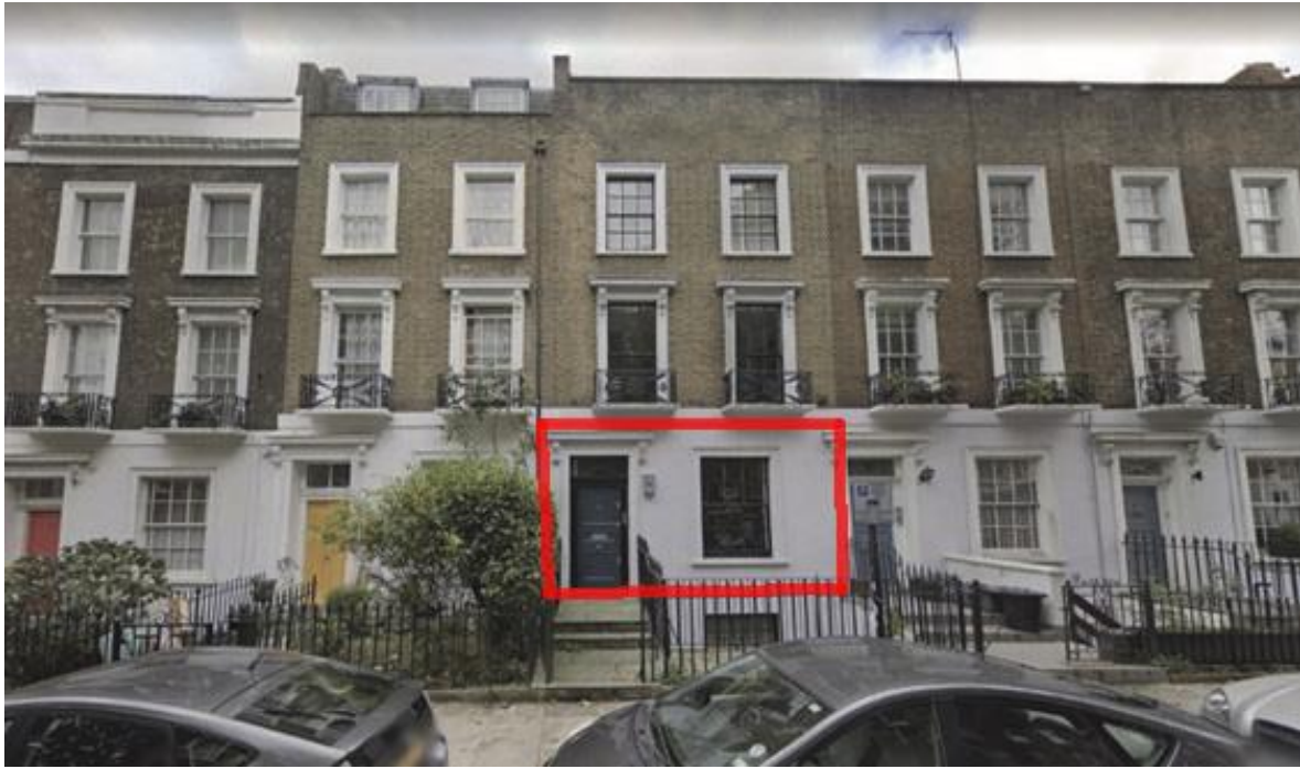
Fig.4 Street view of Arlington Road
