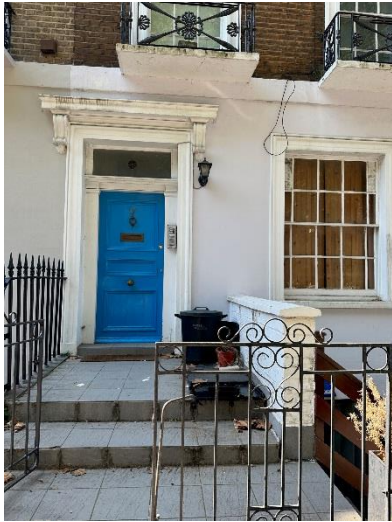
Fig.12 Arlington Road street view
